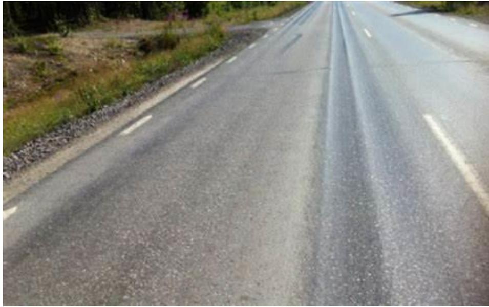
*Figure 2.4: Rutting pavement (Piotr, 2021)*
