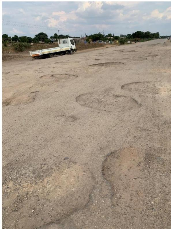
*Figure 4.1: Chitungwiza road severely damaged with potholes, lorry navigating on sidewalk (Source: Author)*
