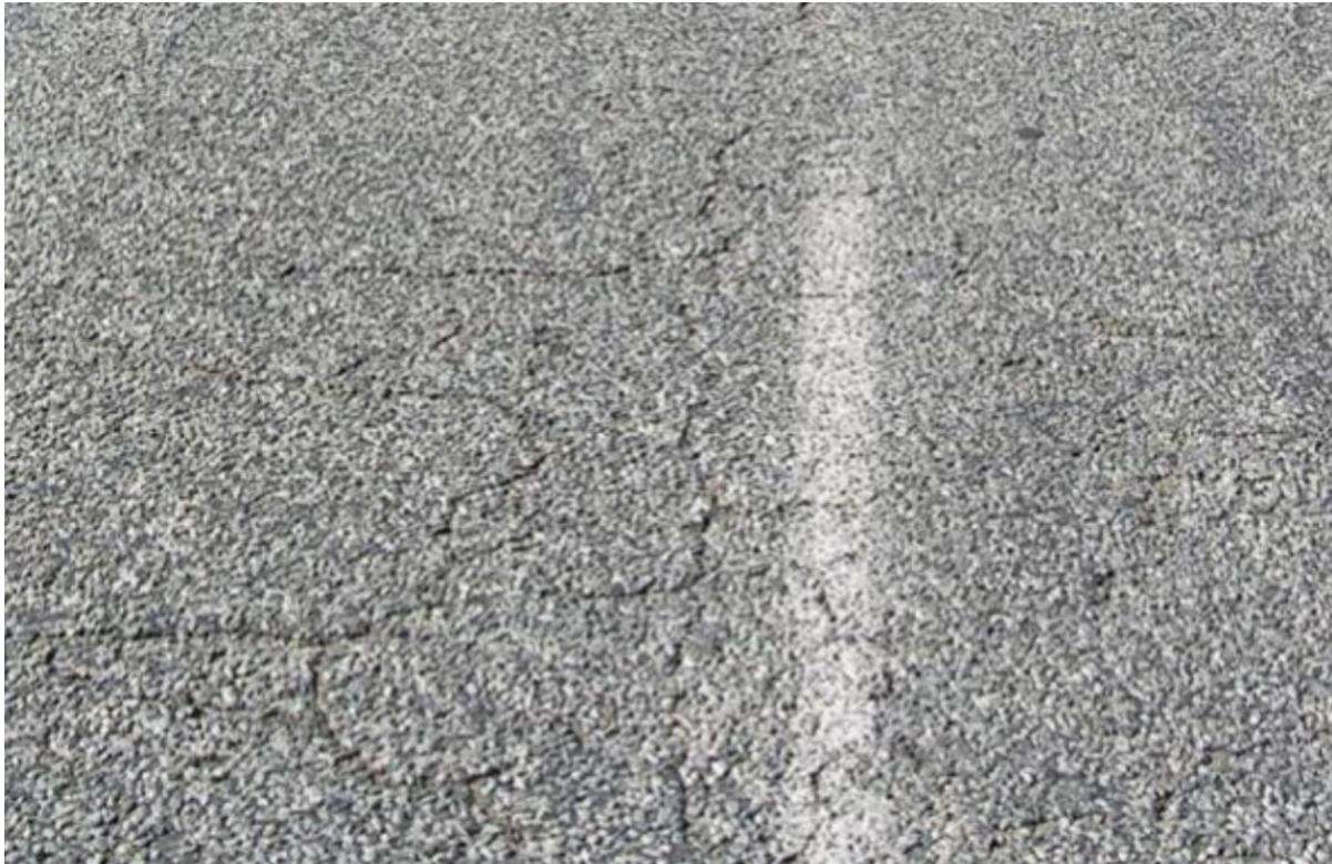
*Figure 2.3: Surface cracks (Pinard & Geddes, 2020)*
